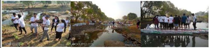
'Shramanubhav'- the fieldwork project aimed at building a dam consisting of around 450 cement bags on the river. Dam was built with the purpose of storing water for local farmers for the summer season. They worked tirelessly 4 hrs. per day from  $31^{\rm st}$
